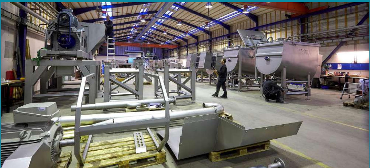
View over scansteel foodtech® final assembly hall.
